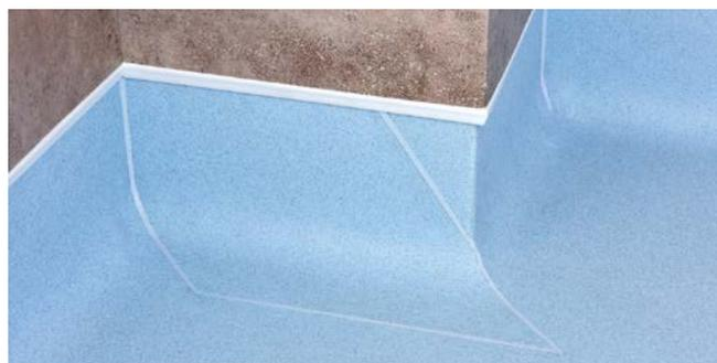
Figure 11 External corners 'wrap around method'
