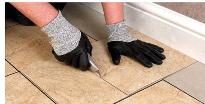
Figure 6 Measuring using an overlapping tile
