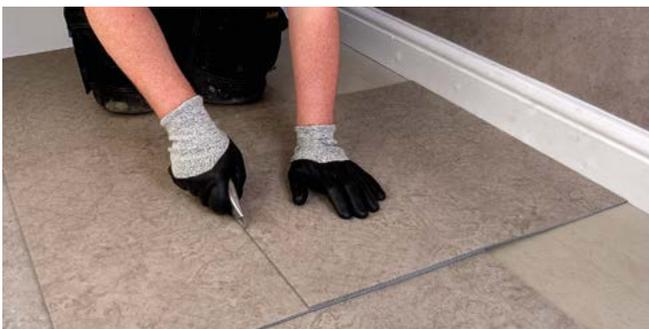
Figure 8 Measuring using an overlapping tile
