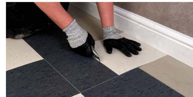
Figure 5 Measuring using an overlapping tile
