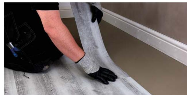
Figure 1 Setting planks out
