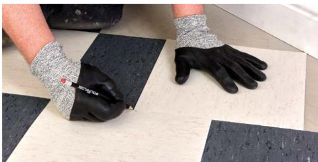
Figure 7 Marking the perimeter tiles (diagonal cut)
