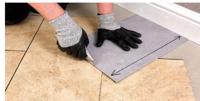
Figure 9 Cutting the perimeter tiles (diagonal cut)
